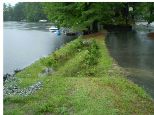
Vegetative swale with rock check dam treats 98% of road runoff to lake
